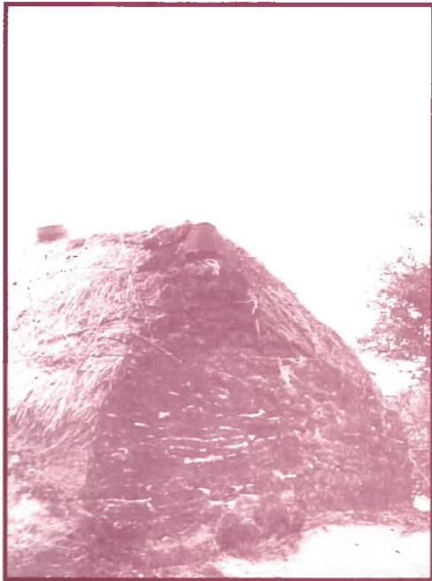
House wall made of sods with marl and mortar in between. Lackan west Wicklow. ( Phoulaphouca Survey, 1939 )
