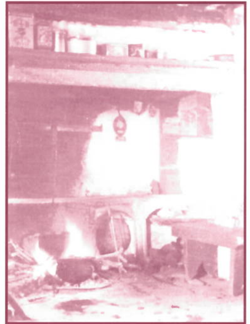
Interior of Class 4 type housing. Notice the fire at floor level with crane and pots. Fuel cavities of carved stone, keepingholes and mantelpiece above.
