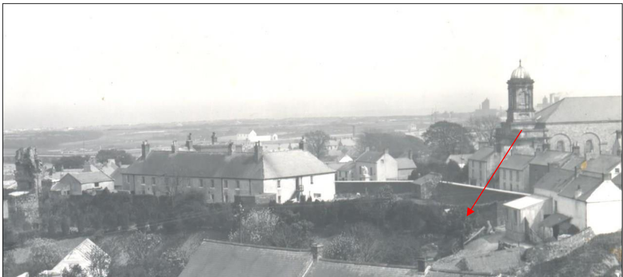
Plate 8: 1899 taken from newly completed St Saviour's church.
