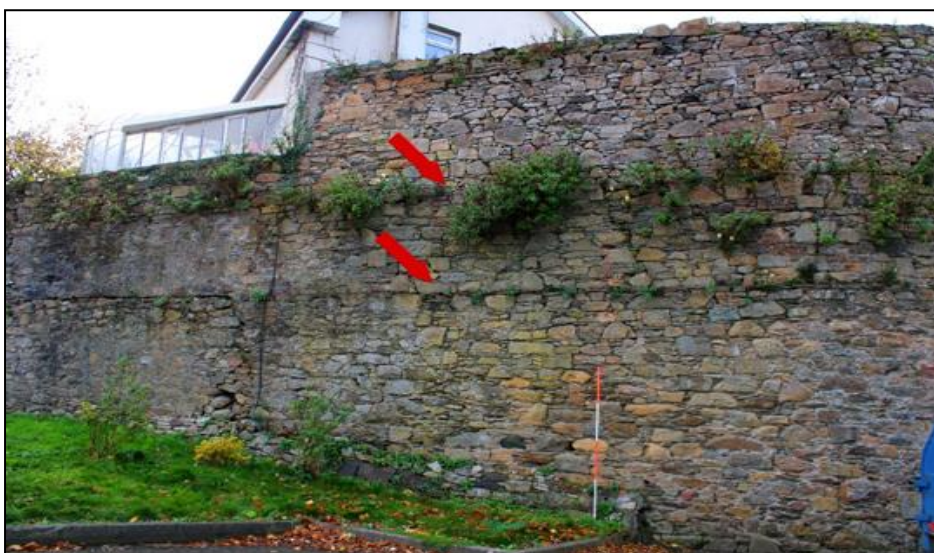
Plate 29: Curtain wall note two phases of construction. The top of the first phase is capped with flat slate stones.
