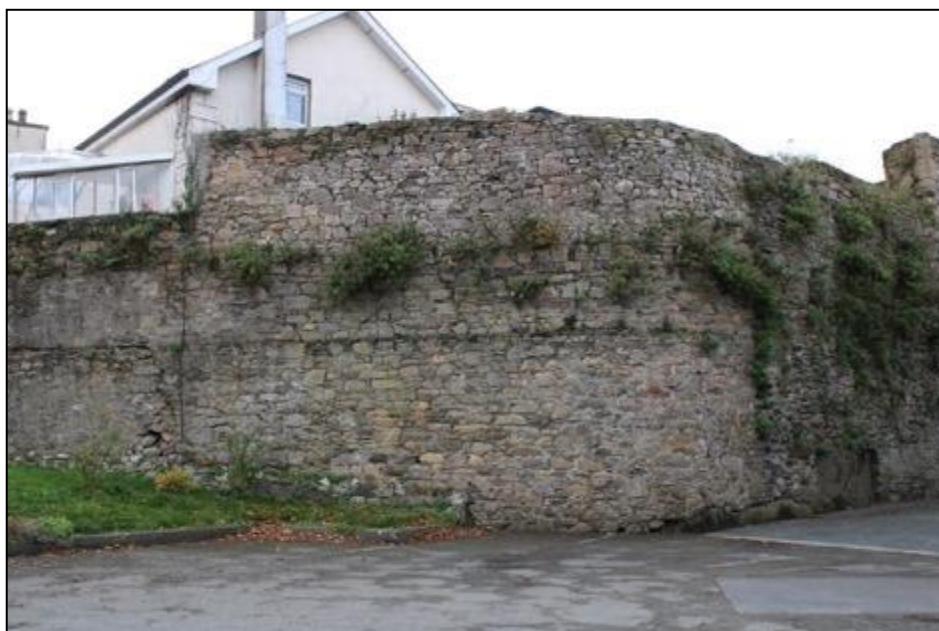
Plate 19: Eastern elevation of curtain wall photo taken facing northwest.
