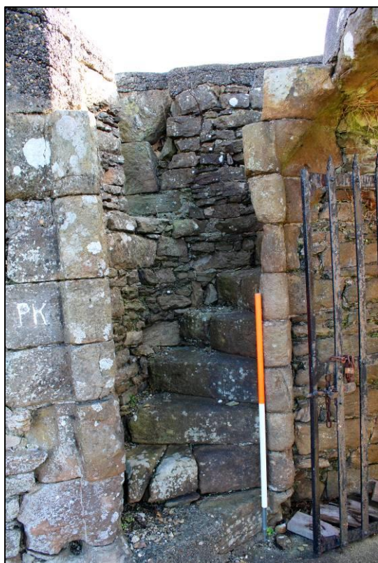
Plate 45: Spiral staircase facing south.
