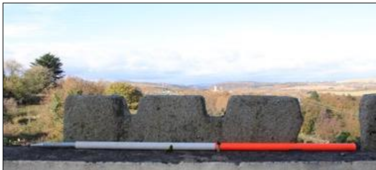
Plate 49: Cut granite stone in grounds of St Anne's.
