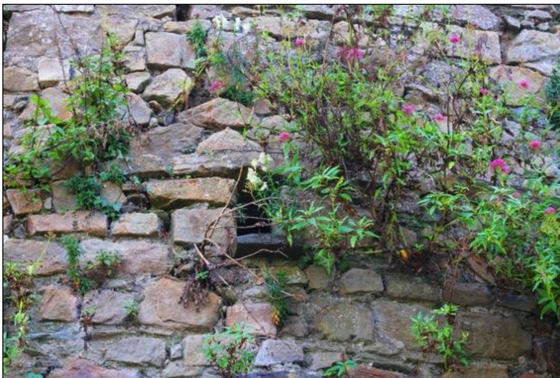
Plate 30: Putlog hole on northeastern elevation of curtain wall.
