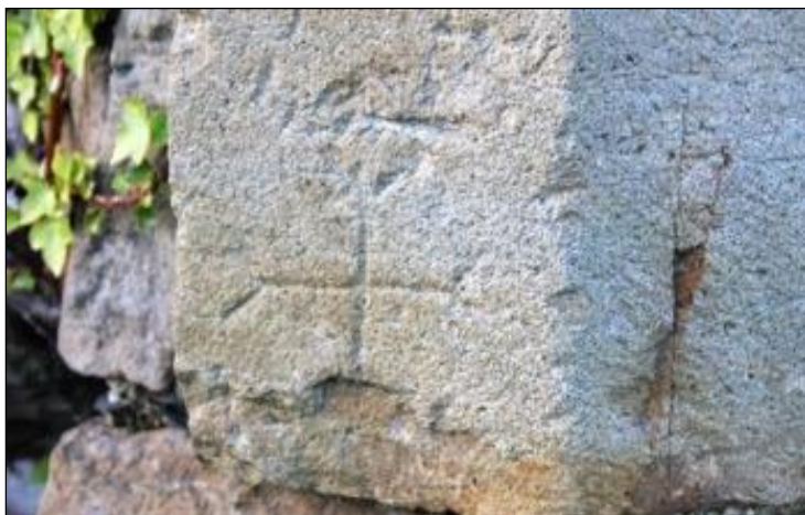
Plate 26: Masons mark at base of window.
