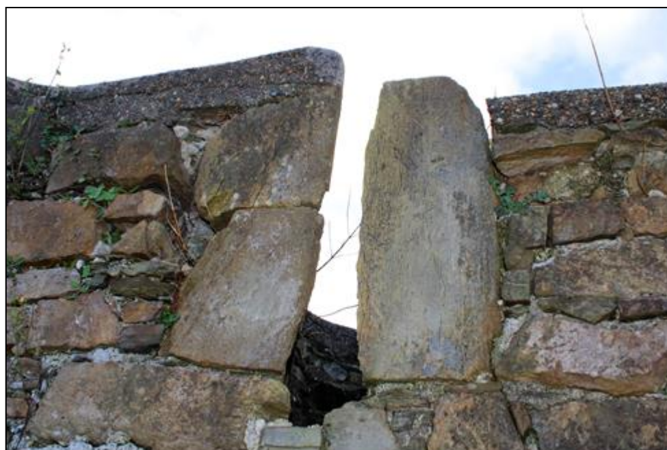
Plate 33: Sandstone splayed arrow slit in tower (see above plate 37 for location).
