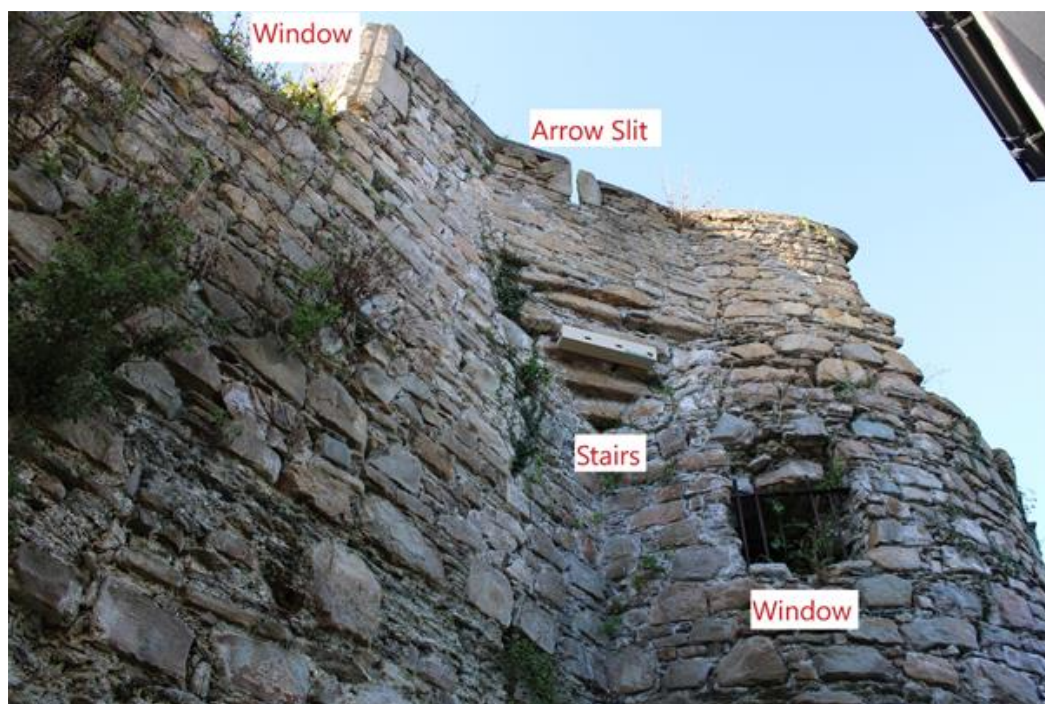
Plate 32: First and second storey of tower with arrow slit on stairs which leads to the no longer extant third storey.
