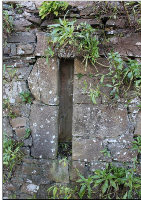
Plate 23: Most southerly arrow slit.
