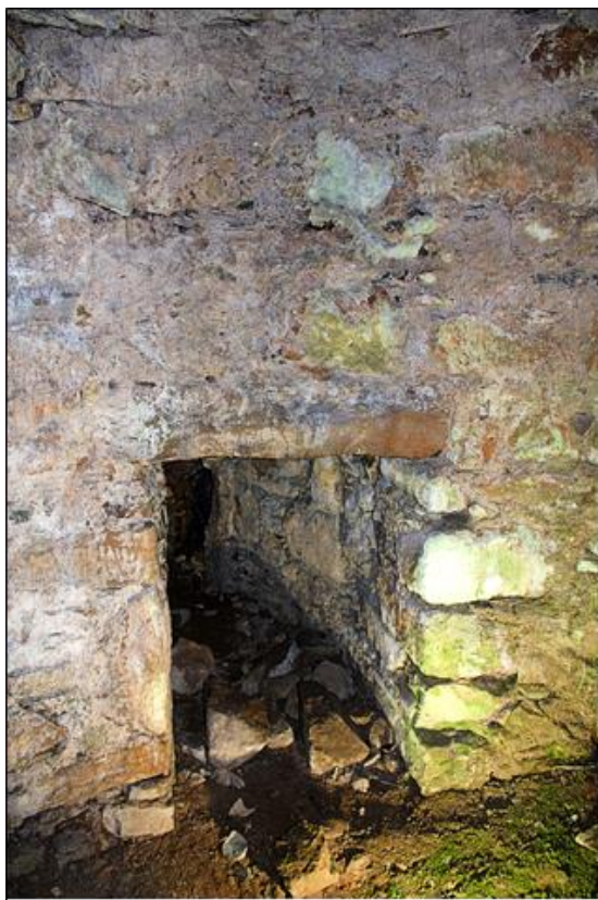
Plate 52: Mural passage in southeast wall of tower, prior to excavation.
