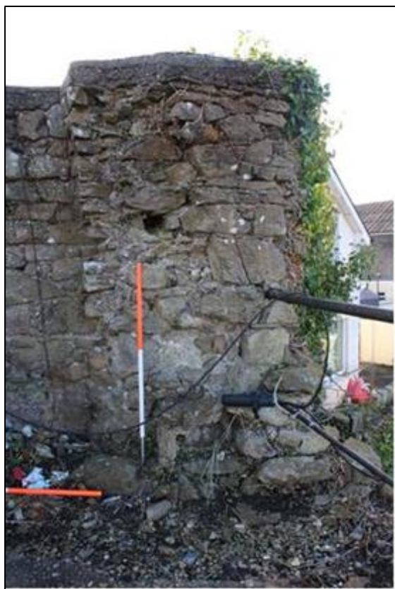
Plate 46: Wall of tower facing south.
