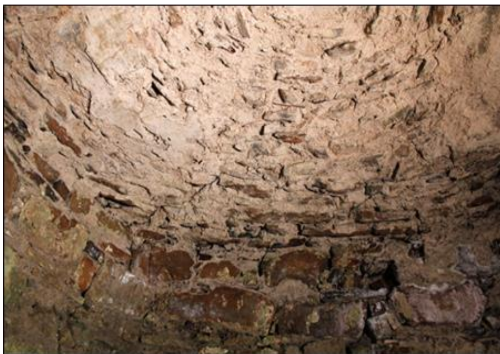
Plate 41: Northern section of soffit within tower.
