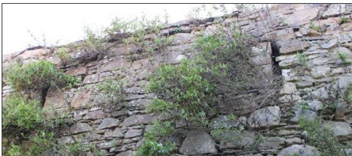
Plate 21: Arrow slits on east facing elevation- arrow slit on right of photo is adjacent to the tower.
