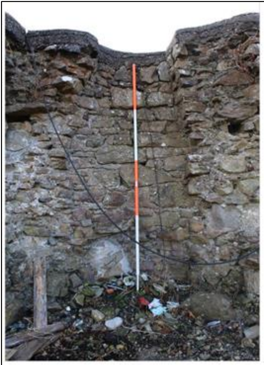
Plate 47: View of possible fireplace in southern wall of tower, facing south.
