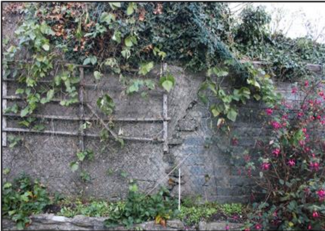
Plate 24: Modern walls built up against section of wall containing arrow slits in the grounds of St Anne's facing east, note original castle wall protruding from cement at centre of photograph.
