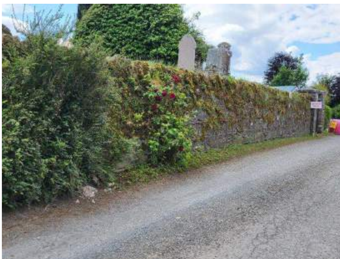
14 North Graveyard wall central section
