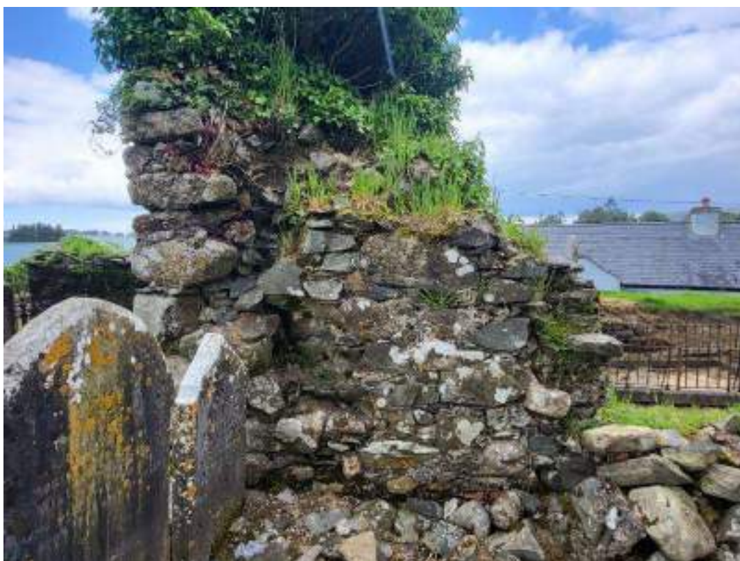
4. Detail of South-West corner (exterior)
