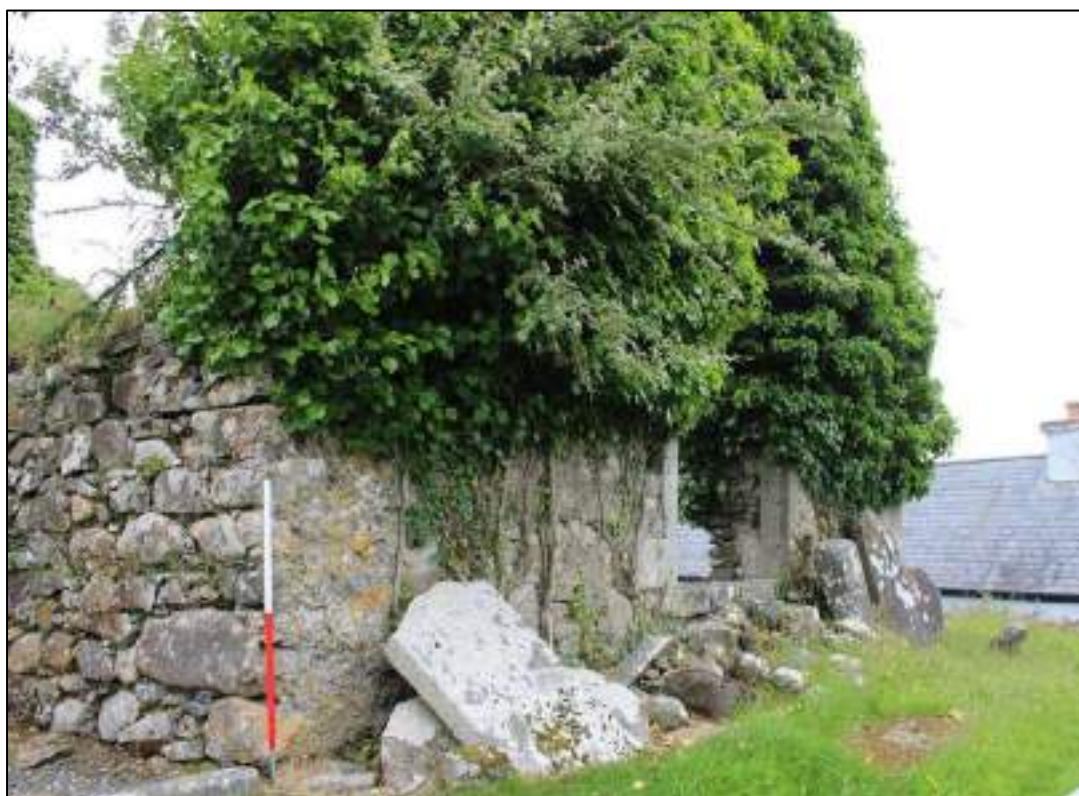
Plate 33: View of southeast corner of eastern gable of the church.
