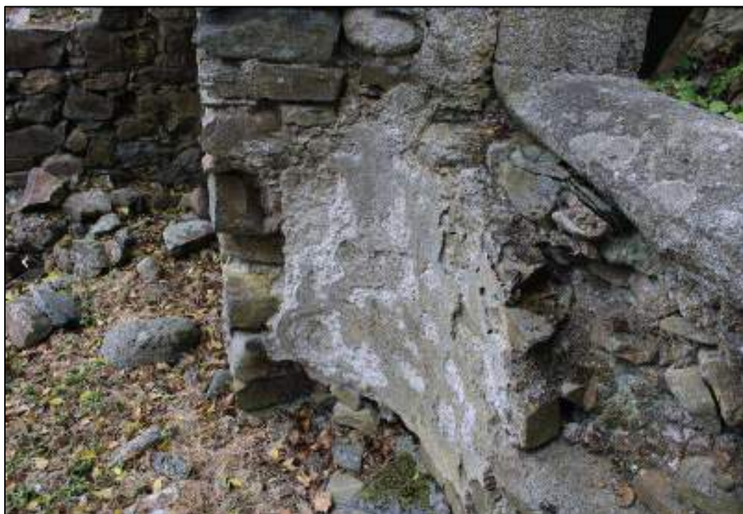
Plate 37: View of plaster below east gable window.
