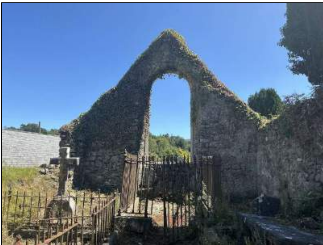
Plate 59: East gable of church with intact granite voussoirs.
