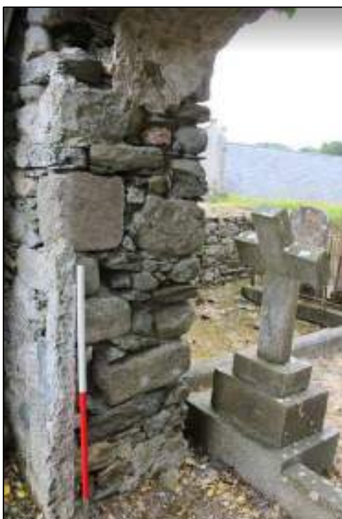
Plate 18: View of northern jamb of the doorway.
