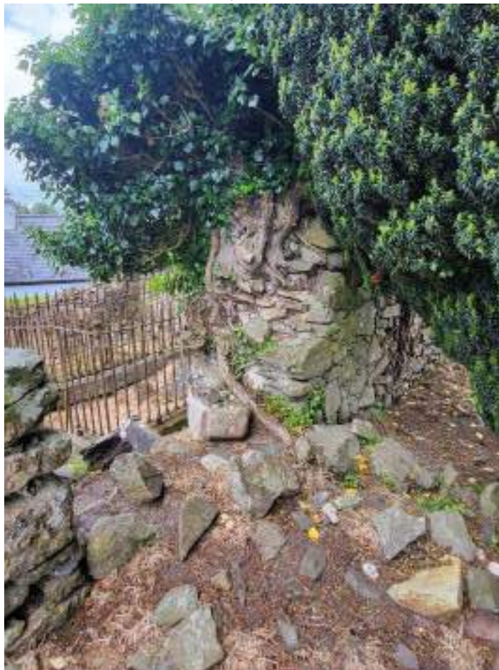
6. South Wall, centre (note partially filled in window)
