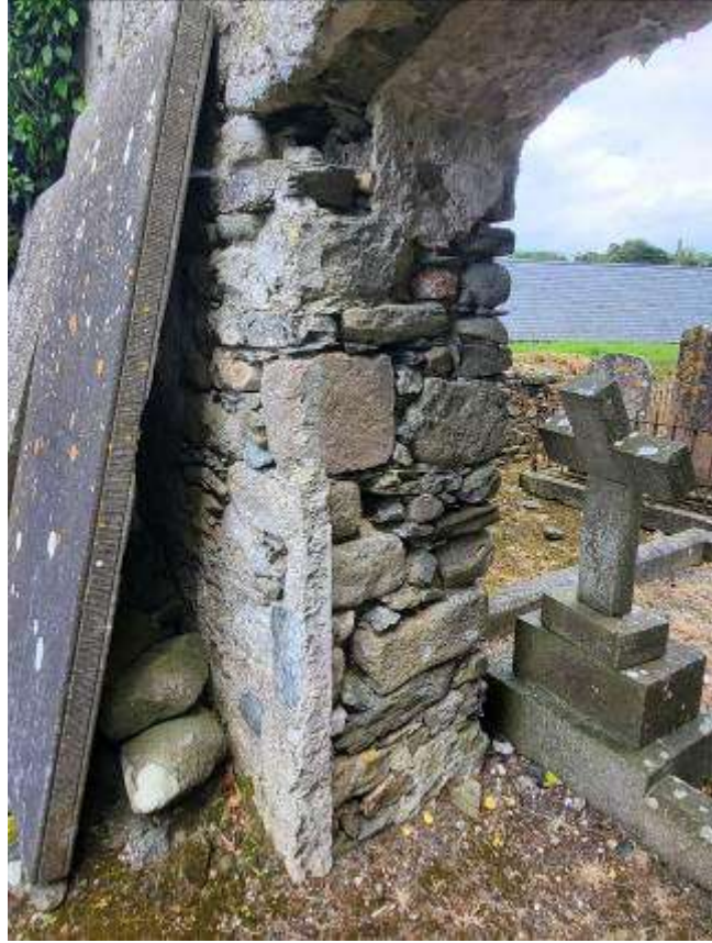
18. Detail of West door reveal (note absence of pointing)
