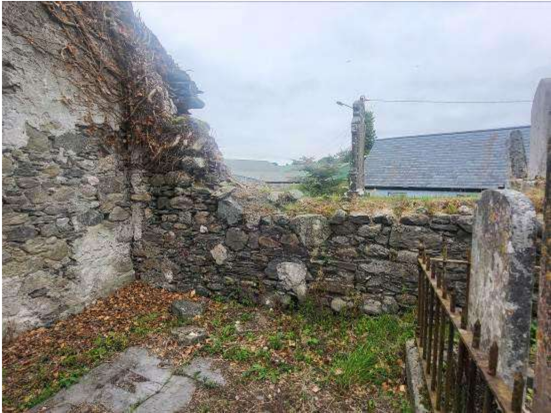
9. North wall interior, west end
