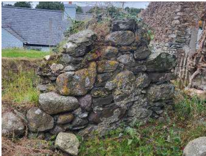
14. South wall remaining central section (external)
