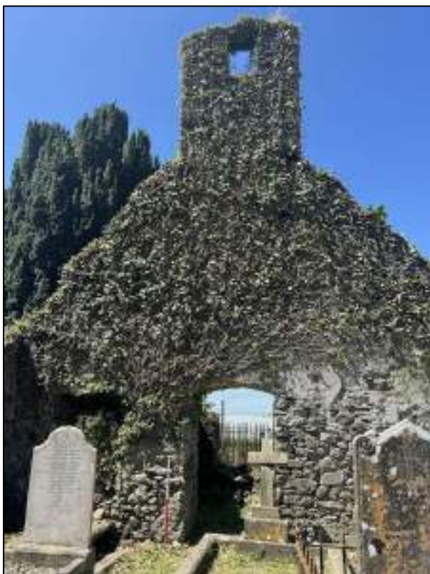
Plate 61: Bellcote in west gable of church and central doorway in west gable.
