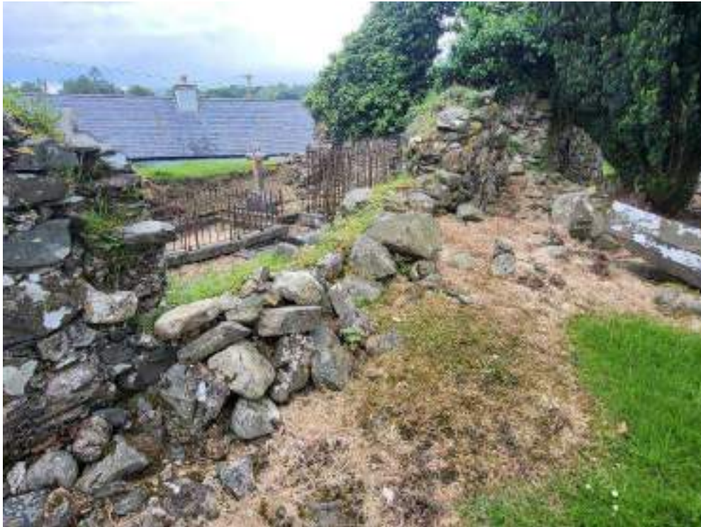
5. South Wall, west end (note window reveal at left side)
