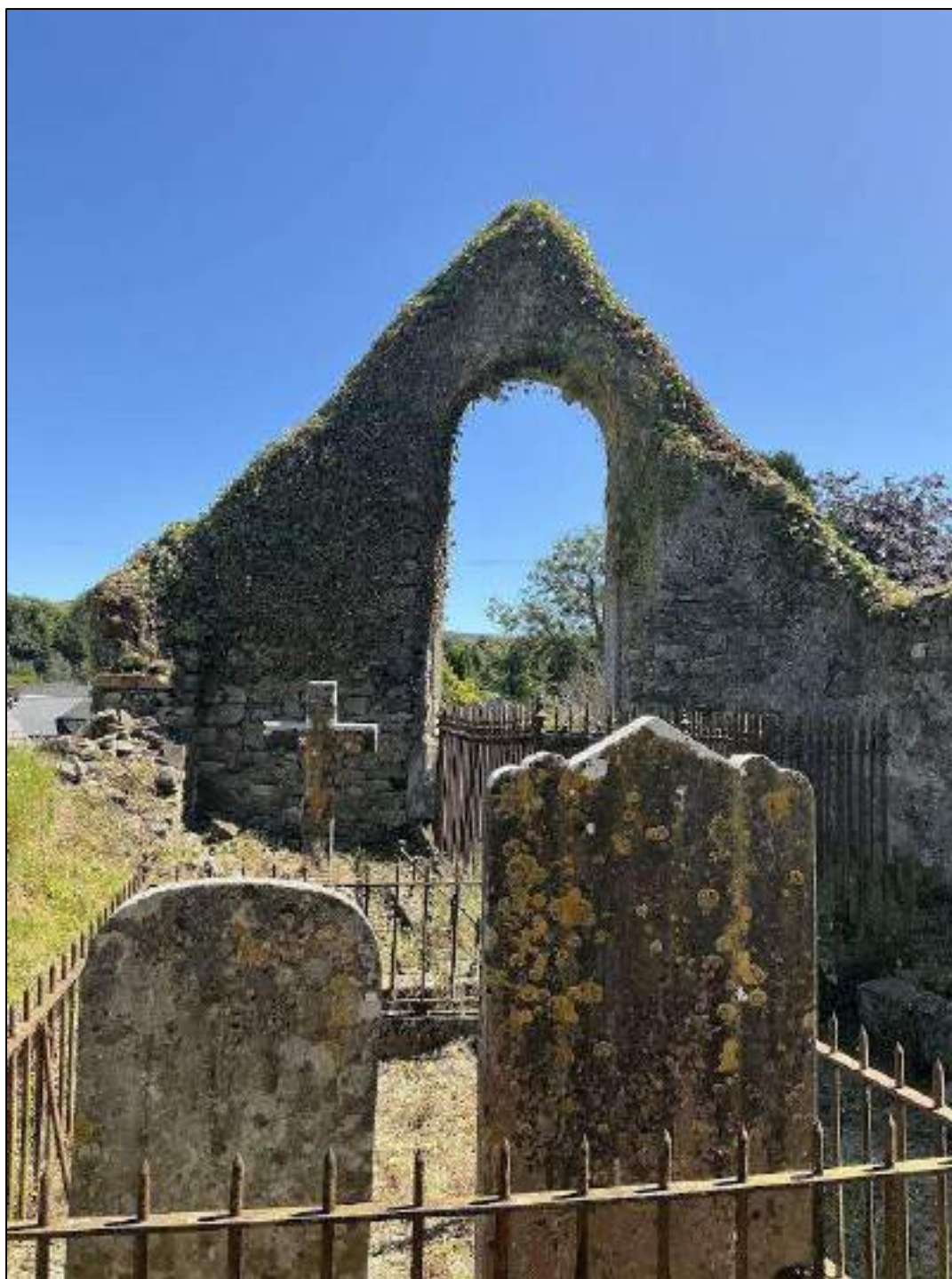
Plate 53: View of east gable from interior of the church.
