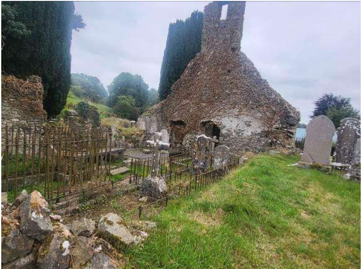
6. West wall interior (Note view of remnant North wall from outside).
