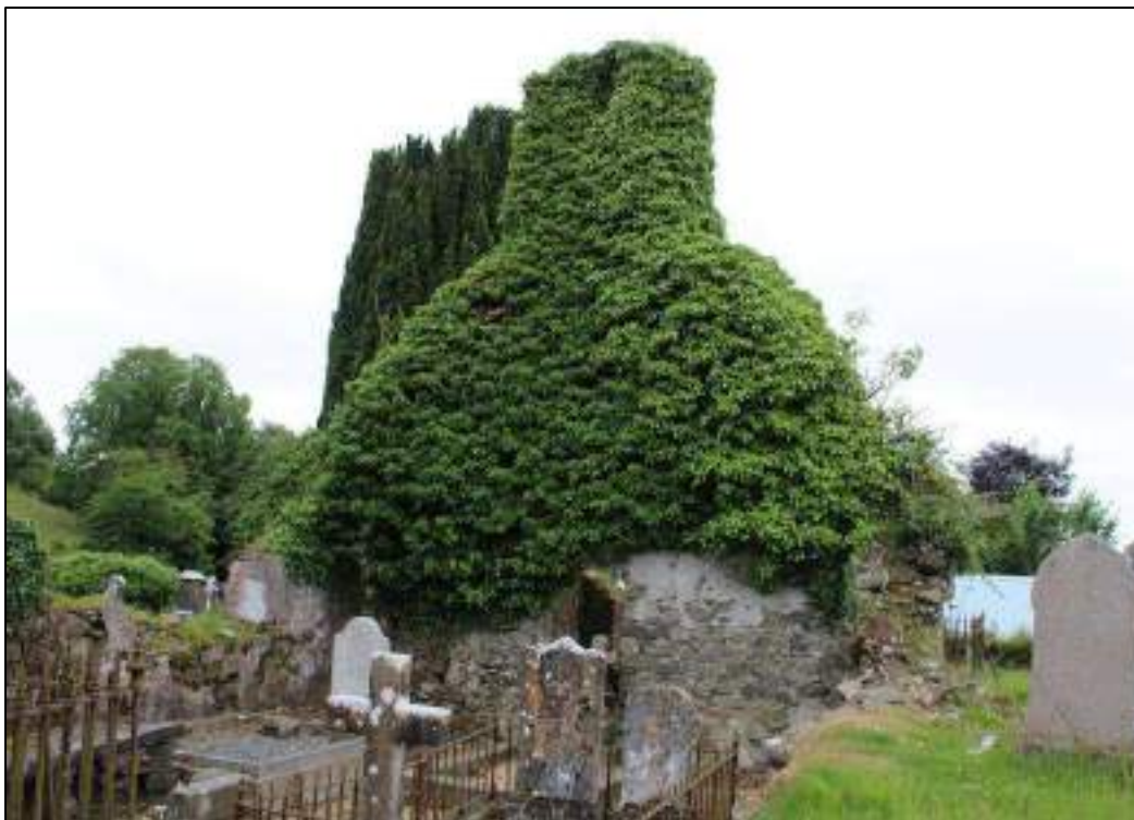
Plate 15: Internal view of west gable, note bellcote and entrance doorway.
