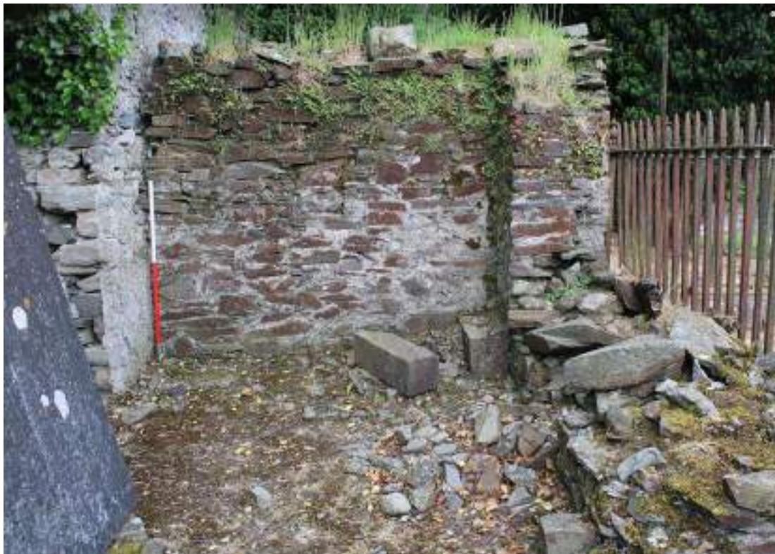
Plate 19: Later wall which abuts the west gable of the church at the doorway.
