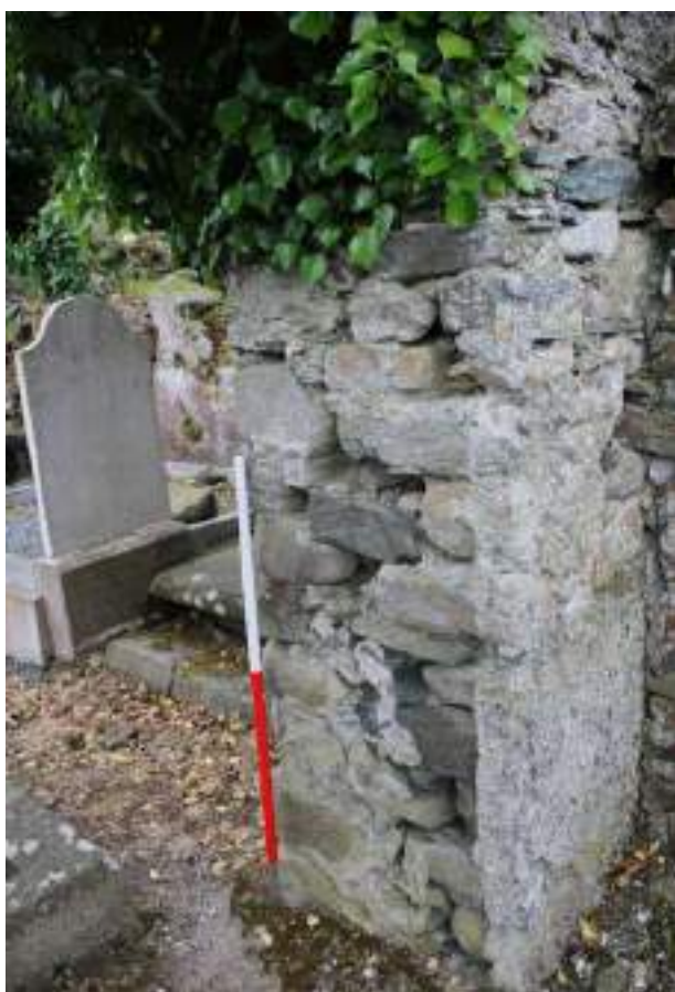
Plate 16: South jamb of doorway.
