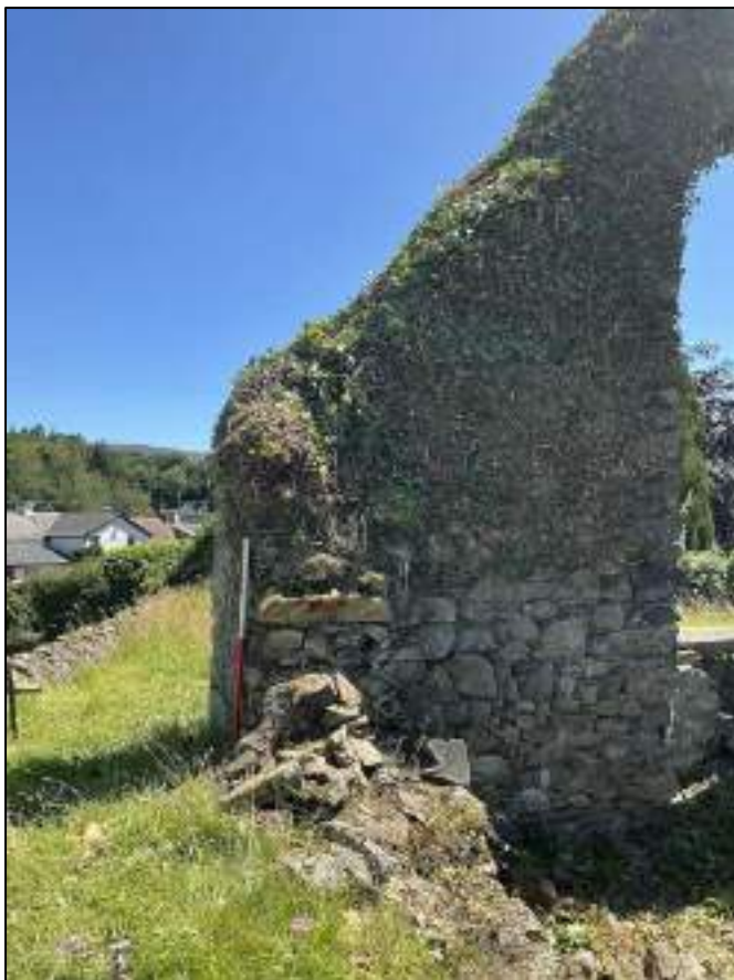
Plate 56: North wall and east gable of church.
