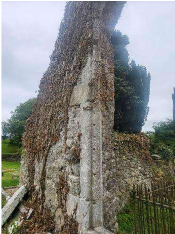
12. Remnant of window detail on ashlar reveal of East window
