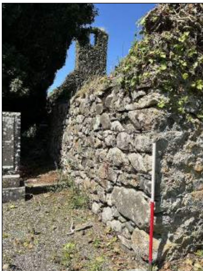
Plate 52: South wall of church and view or bellcote.
