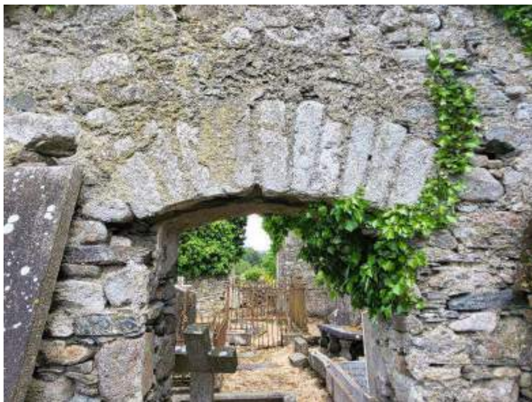
2. Detail of arch in West Wall
