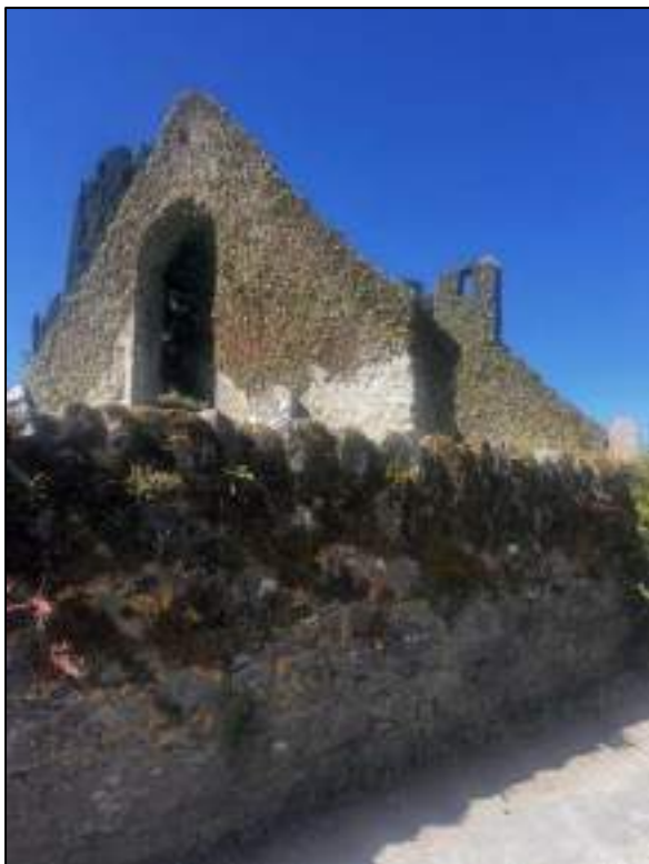
Plate 64: View of church from village towards east gable wall.
