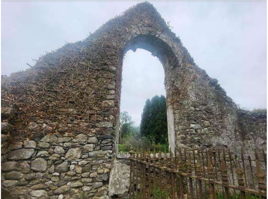
2. East wall interior
