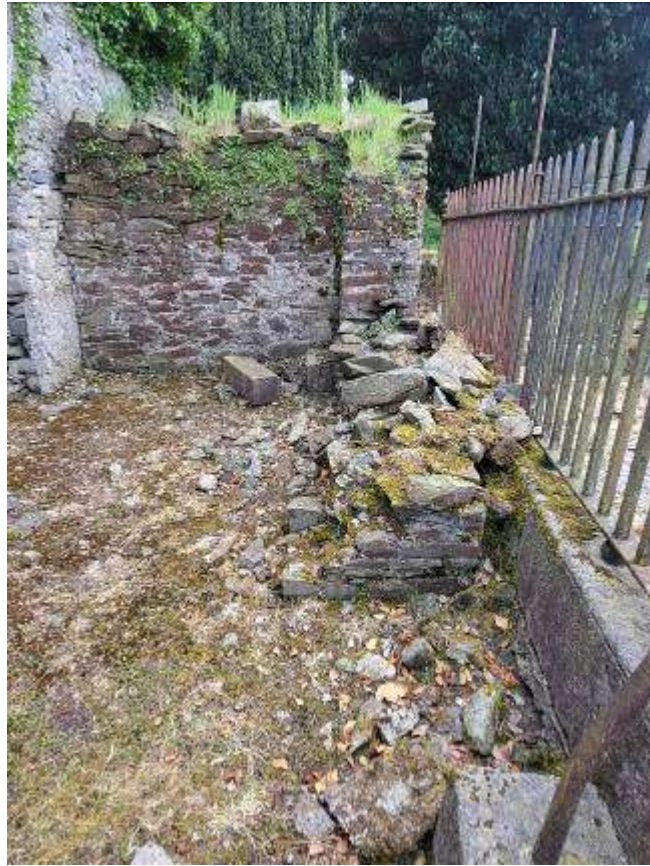
16. Former South porch wall at the west end of the church
