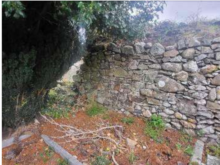
13. South wall East end (external)
