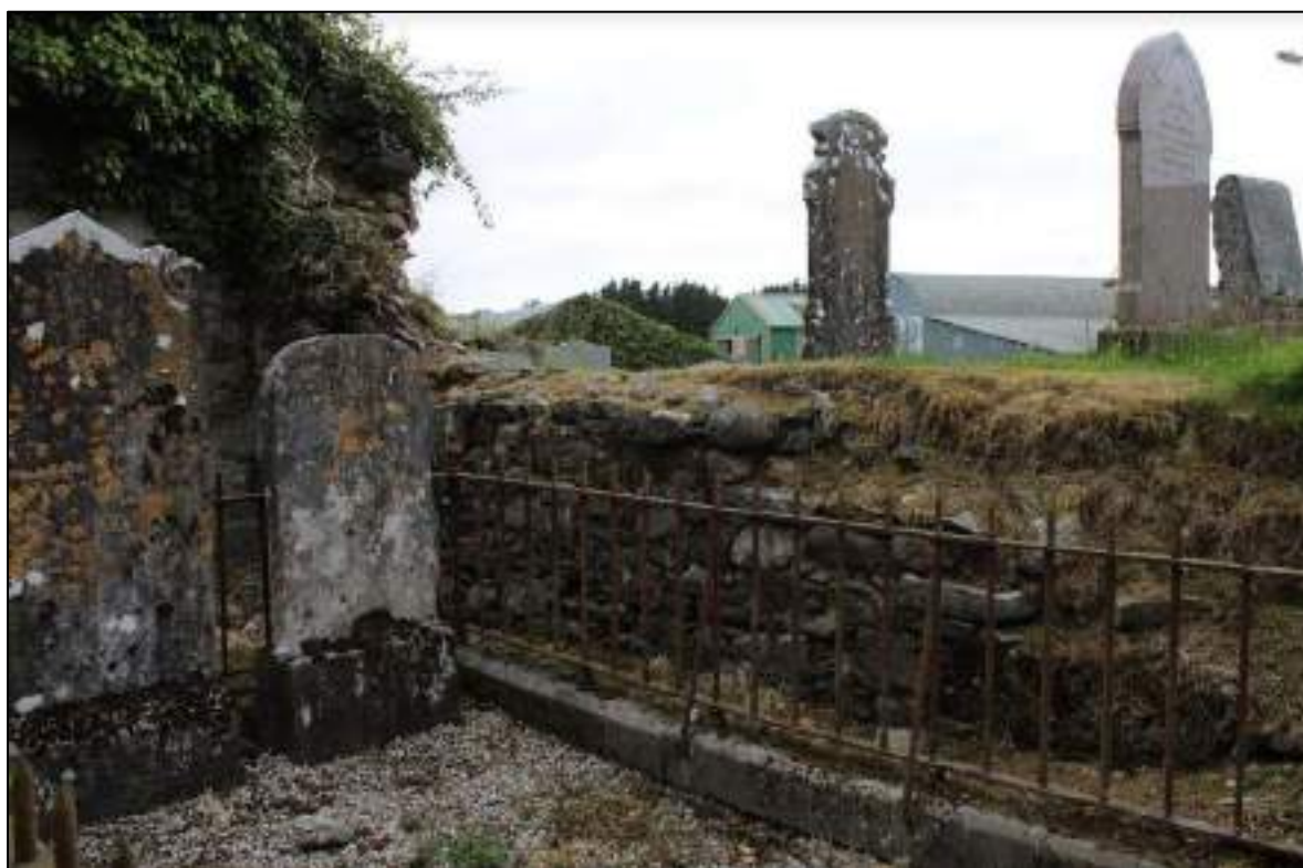
Plate 38: North wall of church and western gable.
