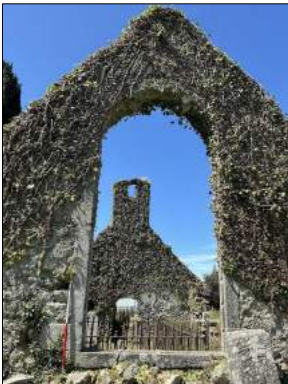
Plate 57: East gable of church and east window exposed.
