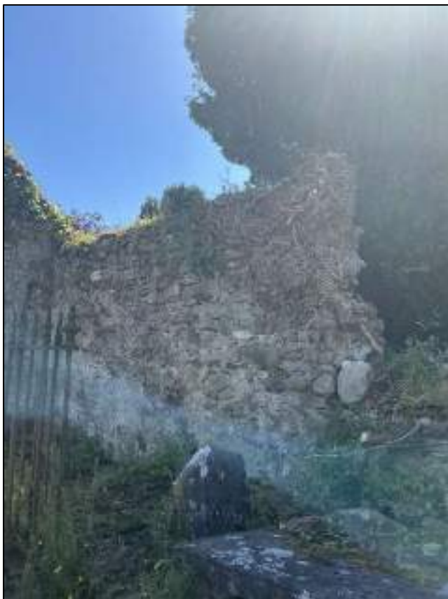
Plate 62: South wall of church and location of window.
