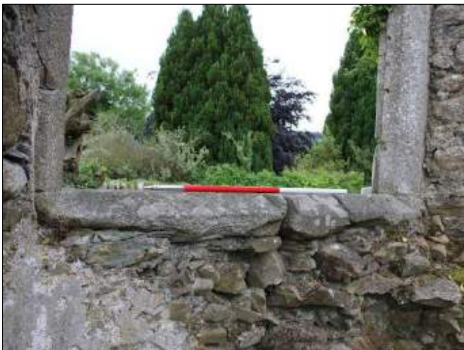
Plate 35: View of granite windowsills from interior of the church.
