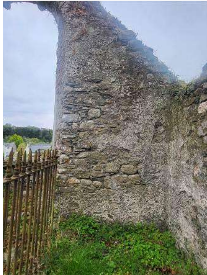
3. Southeast corner internal
