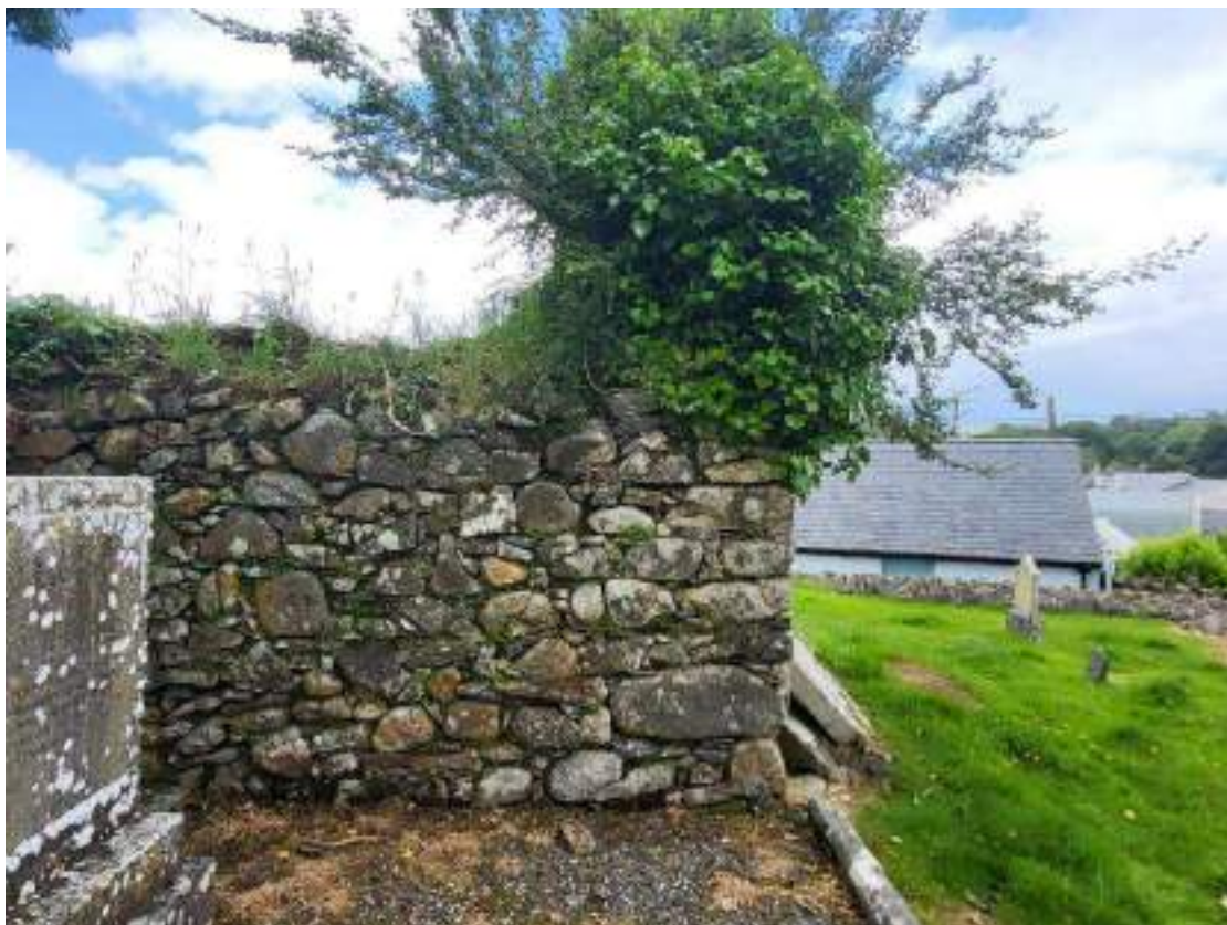
7. South Wall, east end
