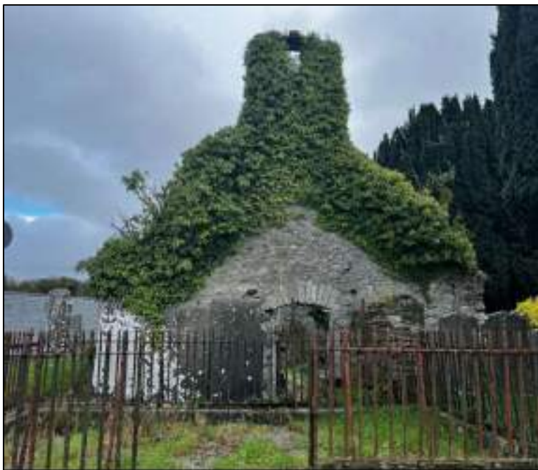
Plate 13: Western gable of the church, bellcote and doorway, the railings in the foreground is the family plot of the Heights.
