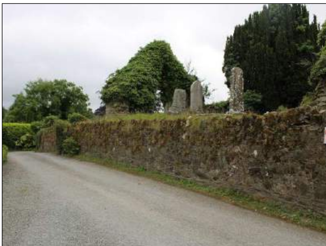
Plate 48: Northern graveyard boundary wall.
