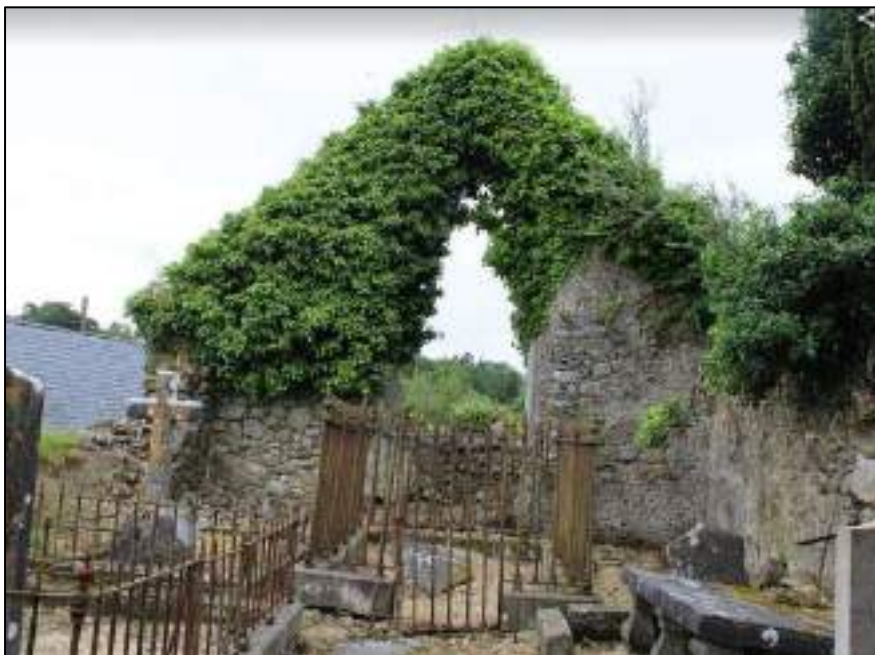
Plate 31: View of east gable window from inside church.
