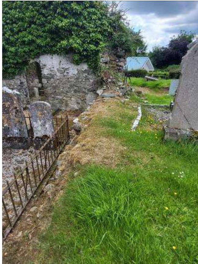
20. Line of the North wall showing raised ground outside.
