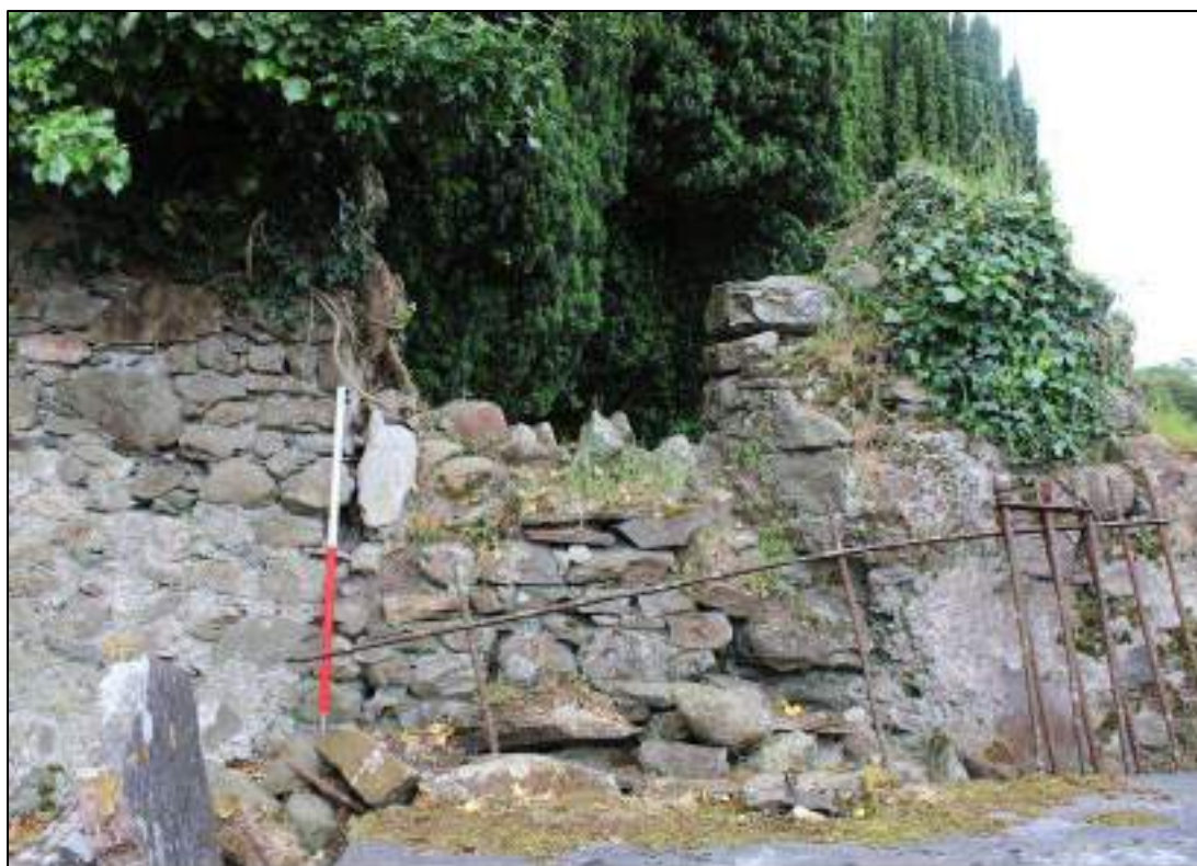
Plate 29: South wall of church with evidence of blocked up window at eastern end.
