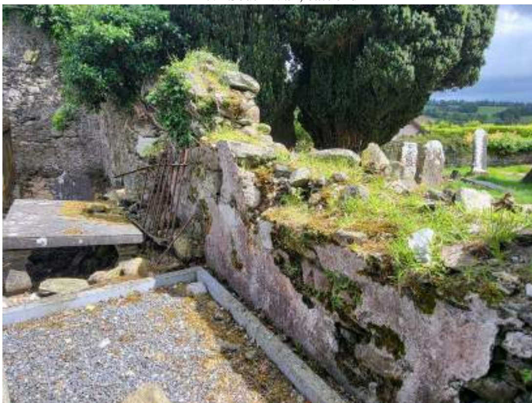
8. South Wall inner face (Note historic plaster)
