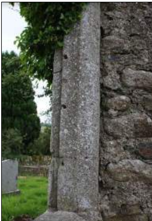
Plate 34: View of granite window jambs with glazing bar holes.
