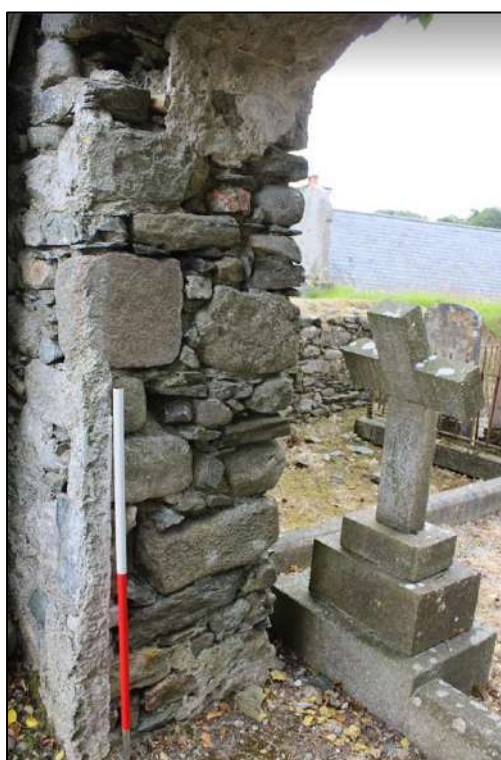
Plate 18: View of northern jamb of the doorway.
