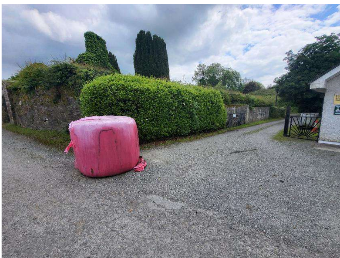
15. West graveyard wall, north end (Note vegetation)
