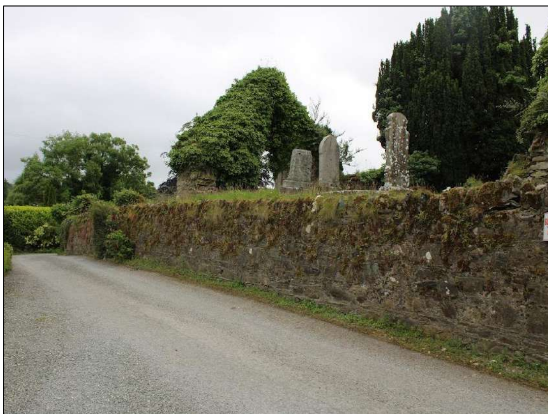
Plate 48: Northern graveyard boundary wall.
