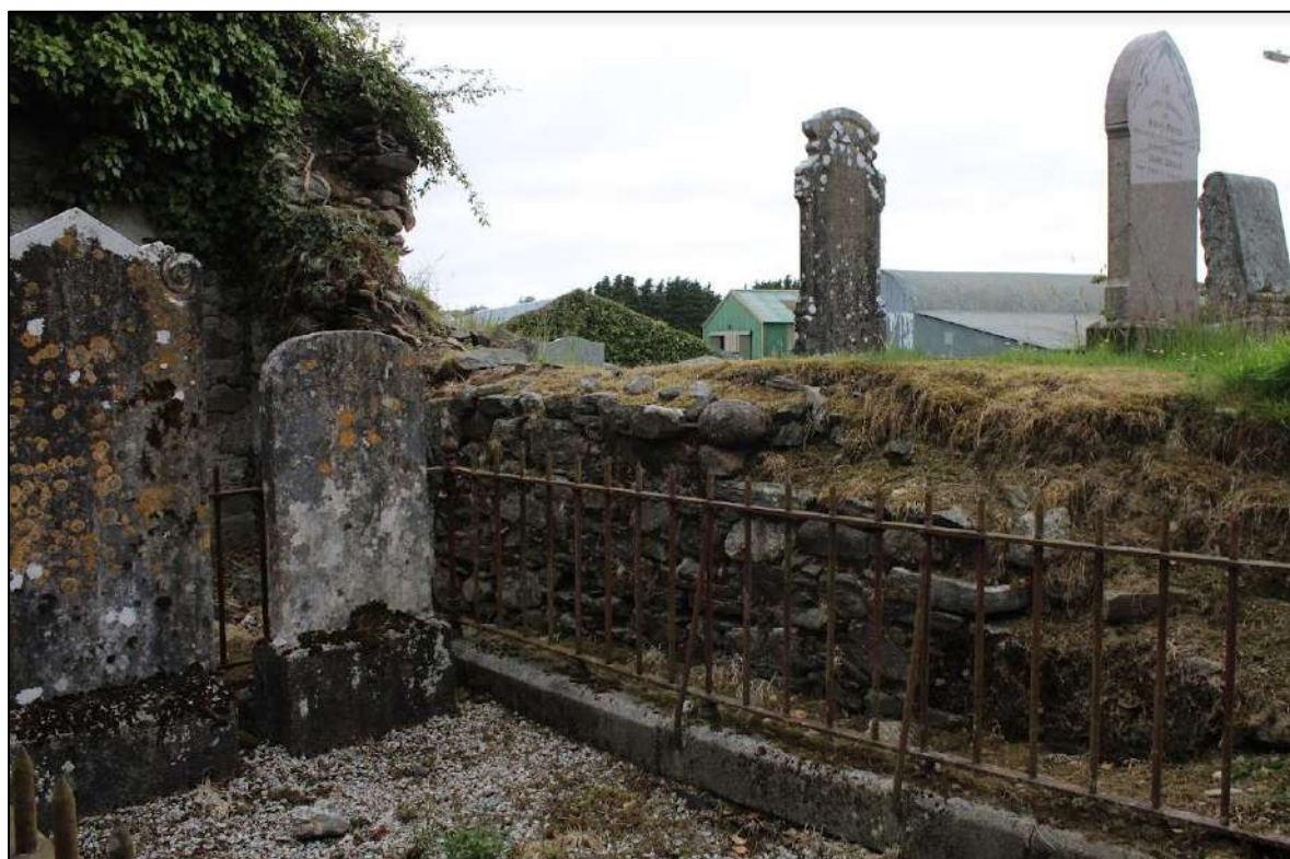
Plate 38: North wall of church and western gable.
