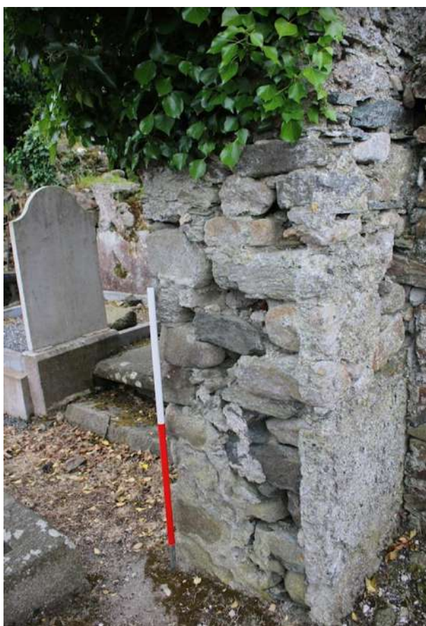
Plate 16: South jamb of doorway.
