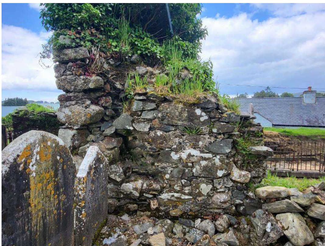
4. Detail of South-West corner (exterior)
