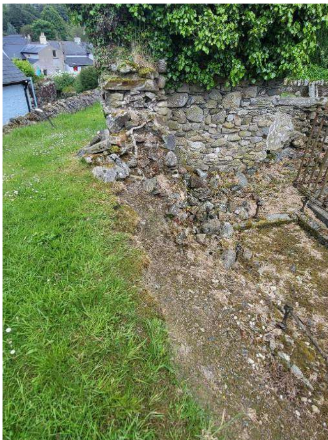
11. East Wall, north end and North wall east end (Note collapsed masonry under windowsill, and earthen bank on the line of the North wall).
