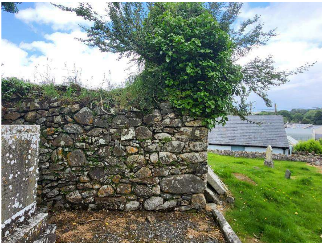
7. South Wall, east end
