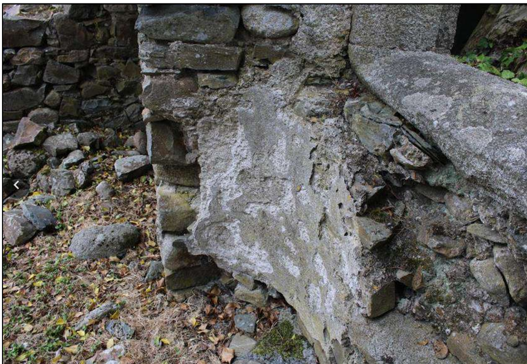
Plate 37: View of plaster below east gable window.
