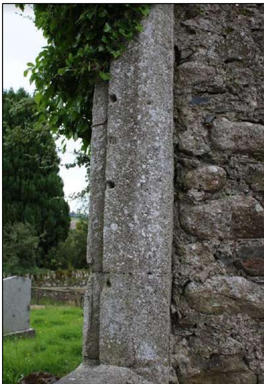
Plate 34: View of granite window jambs with glazing bar holes.
