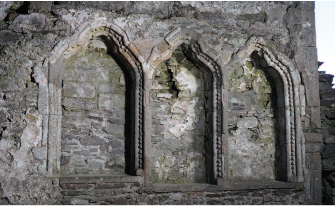
Left: Fig. 9—Thirteenth-century sedilia within the chancel.
