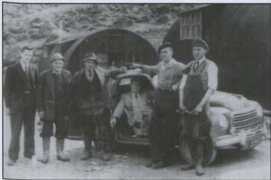
Workers outside Compressor Shed
