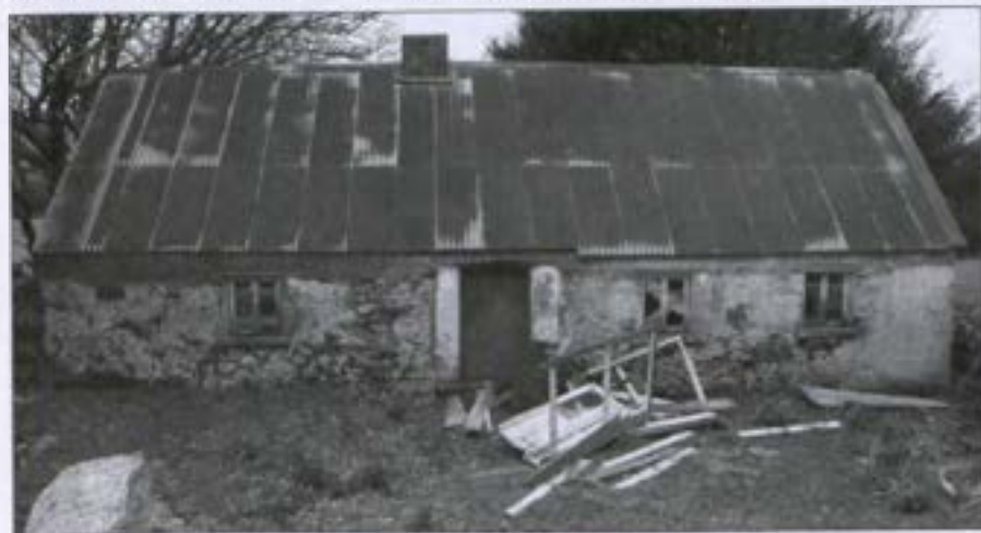
Fig 1 - Abandoned farmhouse at Castlekevin.
