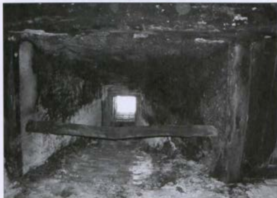
Fig 3 - Looking up a wicker and clay canopy over a fireplace at Castlekevin.
