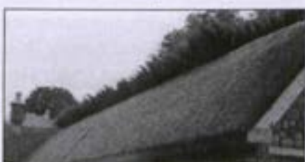
The untrimmed reeds of the ridge
