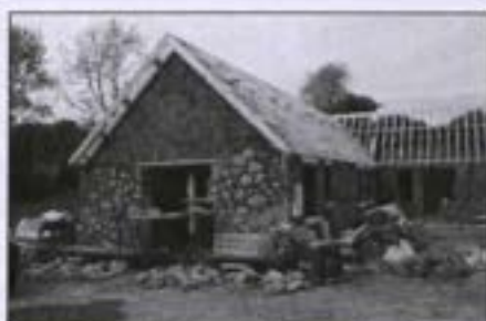
The Start of the Roof
