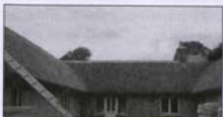
Roof thatch of wheaten straw
