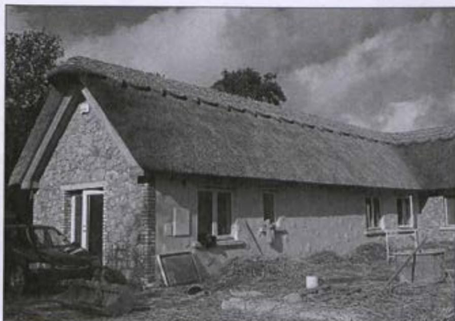
The finished roof
